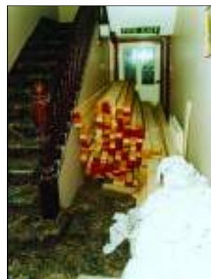
Figure 9: A blocked corridor with incorrect signage
