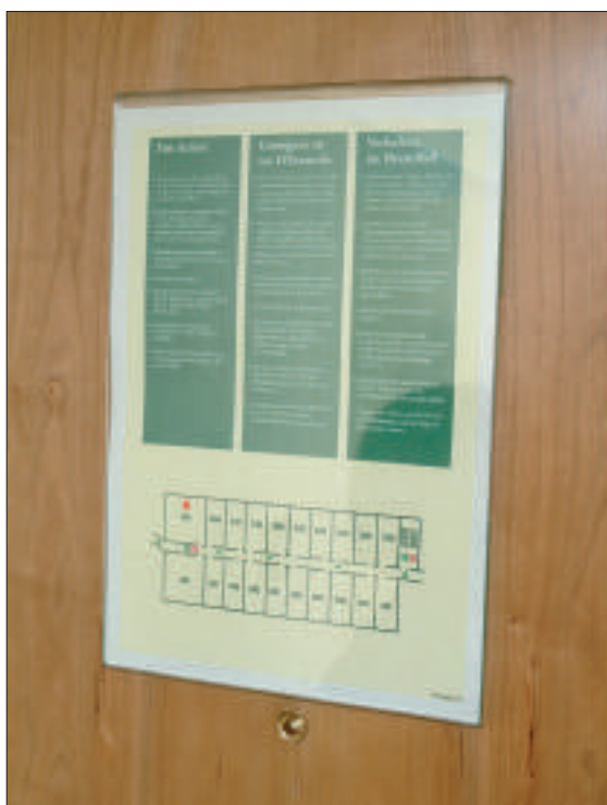
Figure 61: A typical bedroom fire action notice
