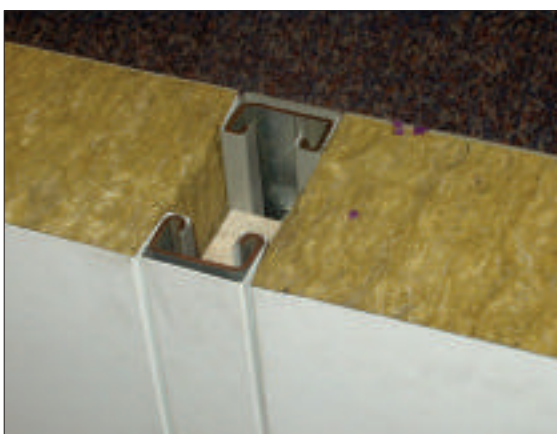
Figure 17: Insulated core panels – internal panel
