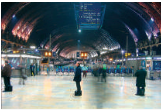
Figure 30: A covered railway station
