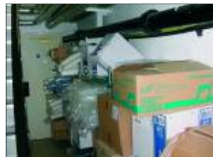
Figure 14: A blocked corridor and exit with incorrect signage
