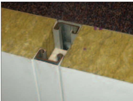
Figure 17: Insulated core panels – internal panel
