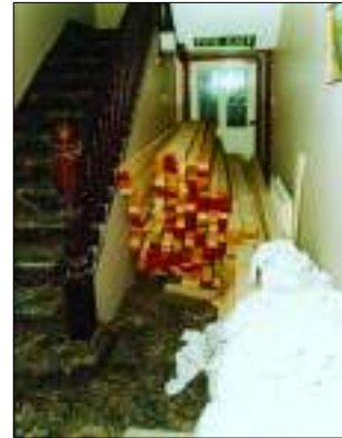
Figure 9: A blocked corridor with incorrect signage
