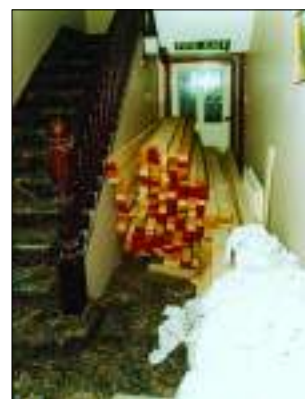
Figure 9: A blocked corridor with incorrect signage
