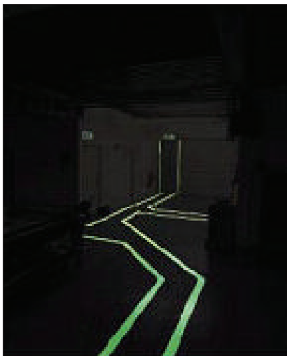
Figure 57: A 'way-guidance' system
